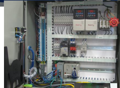
VPN router device mounted inside control panel on Fusion machine.
